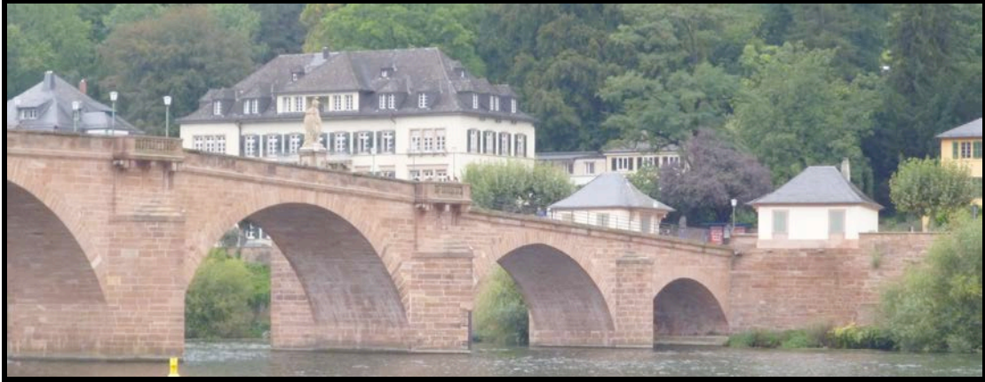
Figure 2. The bridge across the Neckar River, discussed by Heidegger (1950/1967). Photo: G. Stahl, Heidelberg, Germany, 2012.
