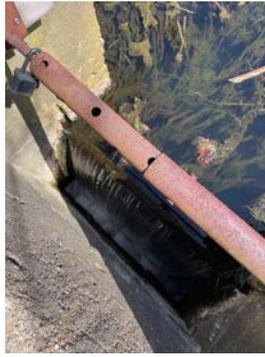
Photo #36 – Two foot water drop in weir from bog to creek
